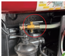
At the Fuel Tank Switch
